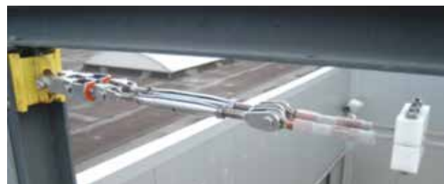
Life Line Tension Indicator for each cable, with Pitchfork, Tensioners & (plastic) Cable Spreader
